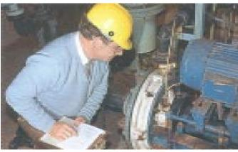
Acid pump, fortified with a C-22 alloy sleeve, is still providing excellent service after 9 years in a continuous stainless steel pickling operation. The acid consists of 2 percent hydrofluoric acid, 20 percent hydrochloric acid, and as much as 40 gm/liter of iron, at 170°F.
